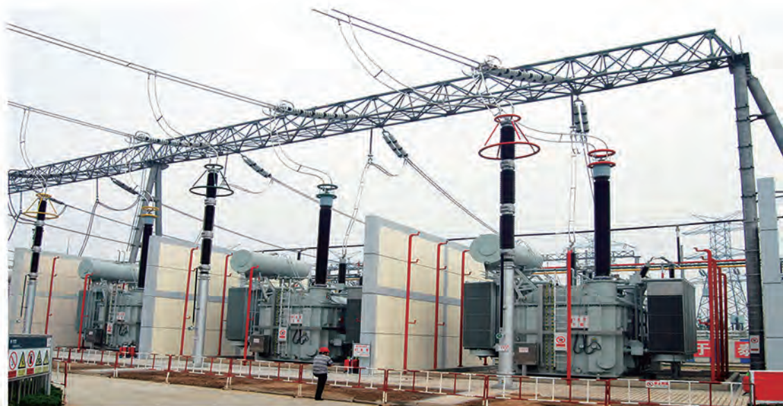
500kV产品安装现场 500kV product installation at site in the transformer station
